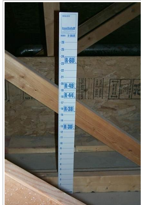
R303.1.3 Insulation Markers Insulation marker installed in attic. Make sure the marker is applicable to the type of insulation installed (fiberglass, cellulose, etc.).
