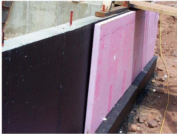
R402.2.8 Basement Walls Exterior insulation R-10 continuous
